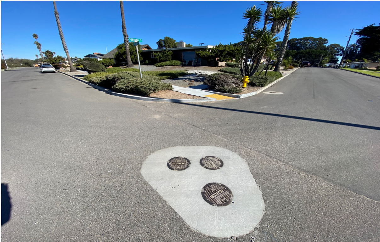
Photograph 3. View of residential neighborhood at southern end of Segment 2-2. View facing northeast. November 17, 2022.
