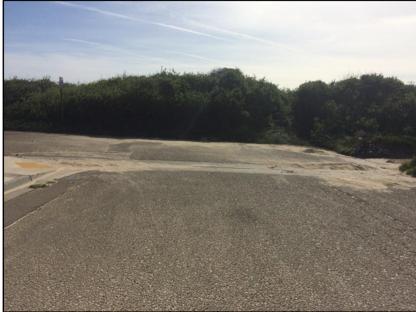
Photo 3. View east of proposed exit pit location on Laguna Drive (April 10, 2018).
