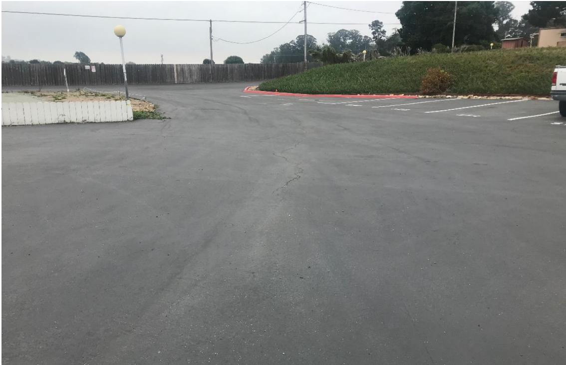
Photograph 5. The BSA within the Ken-Mar Gardens Mobile Home Park parking lot, facing southwest on August 22, 2023.
