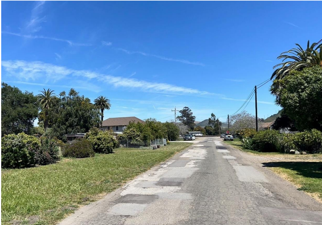
Photograph 9. The BSA at La Due Street and Hiawatha Lane, facing east.
