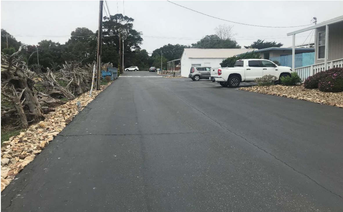
Photograph 3. The BSA within the Ken-Mar Gardens Mobile Home Park driveway, facing west on August 22, 2023.
