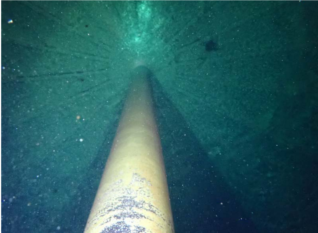
This shot was taken looking upward at the center column. All coatings on the column were in fair condition and no significant corrosion was present.
