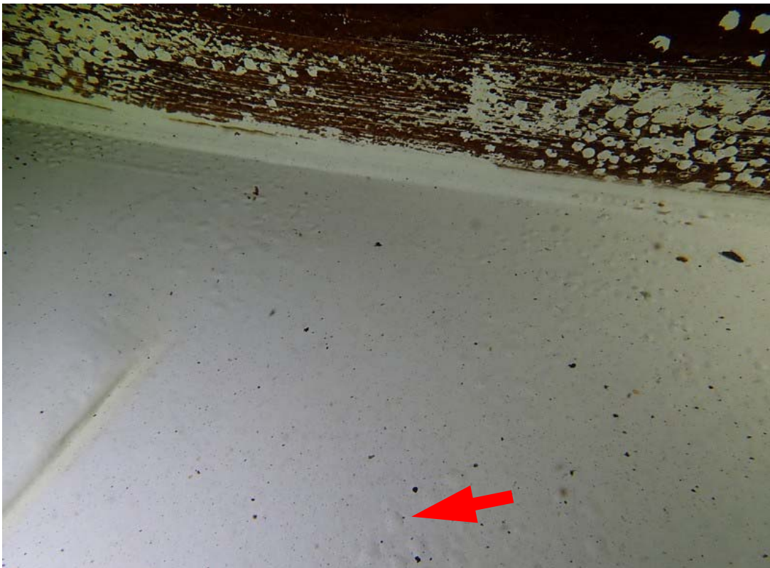
This photo provides a close view of the area shown in the top photo this page. Some scattered blistering is visible (arrow) but no significant corrosion is present.
