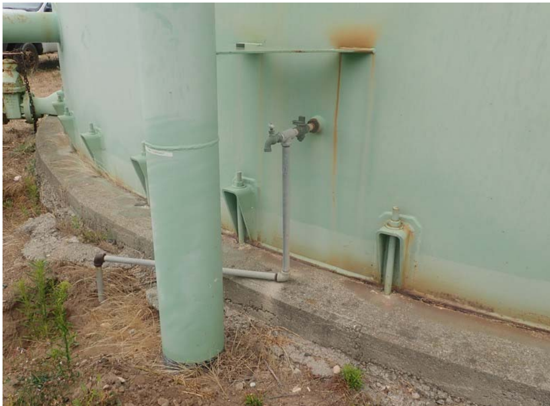
This view shows the existing inlet piping.
