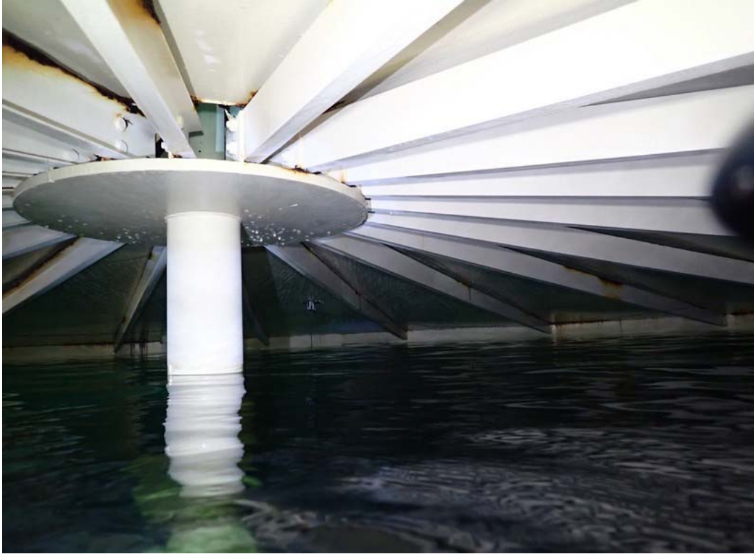
Upper center column, rafters and roof plate.
