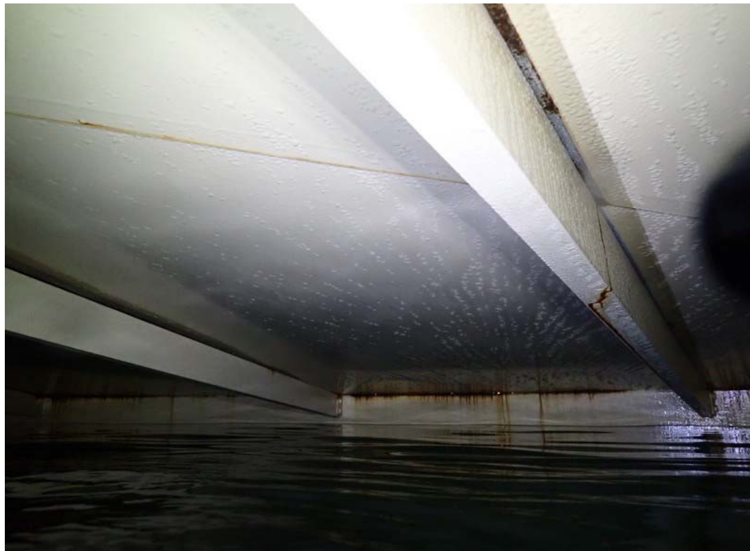
An additional view of the interior roof.
