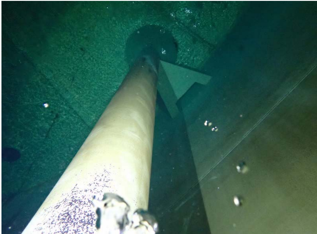
Overflow piping and support as viewed looking upward from the bottom.
