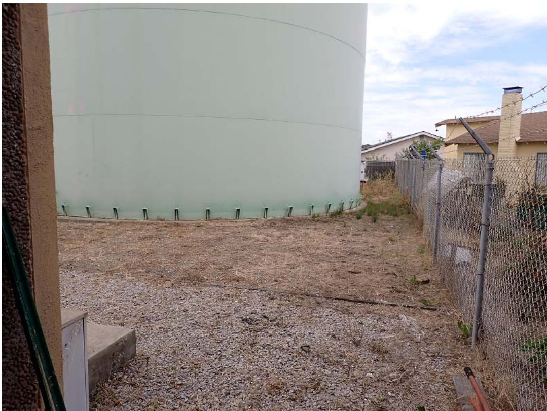
View of site looking northward along the eastern fence
