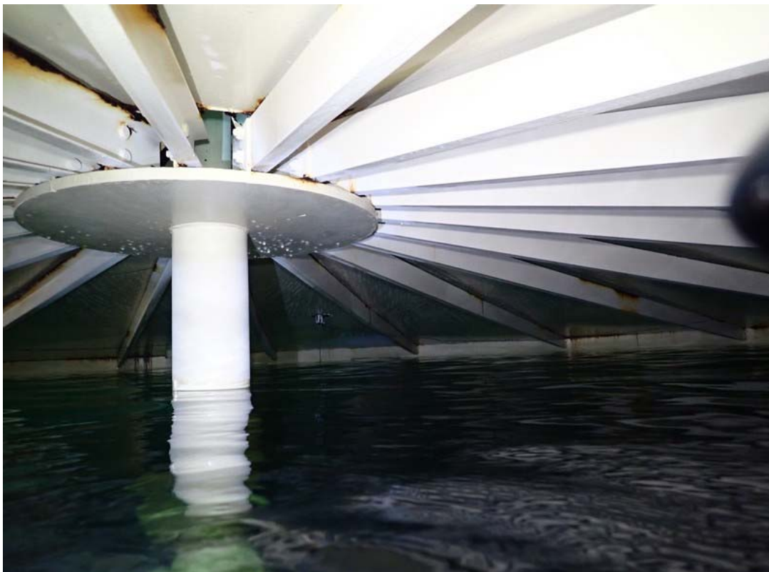
Existing roof column, roof structure and plate that are to be replaced with new formed plate roof.
