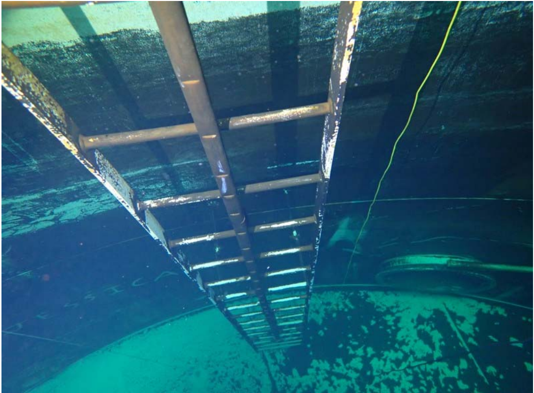
This view shows the interior ladder below the surface.
